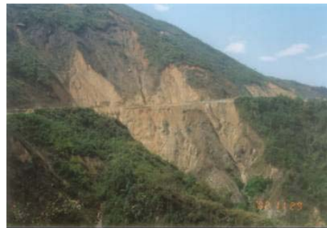
Fig.5 Example of numerous, multiple slope failures triggered above and below the newly constructed highway in Ecuador
