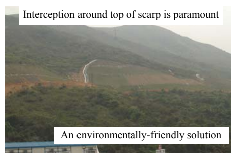
Fig.22 Example of a recent, environmentally-friendly designed back-slope in Hong Kong
