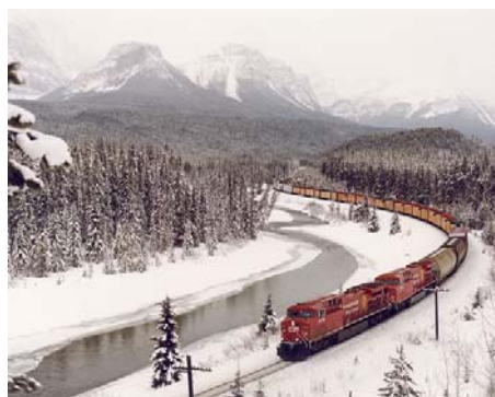
Fig.31 Railway embankments in Canada stretch for thousands of kilometres with failures often producing derailments. Role of soil mechanics in slope stability risk assessment along railway
