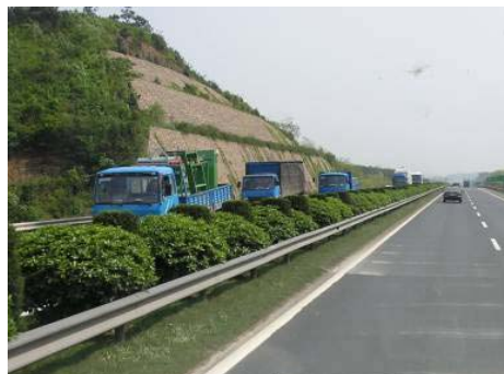
Fig.1 Example of a well-designed highway back-slope on the Hangzhou to Nanjing Highway, China
